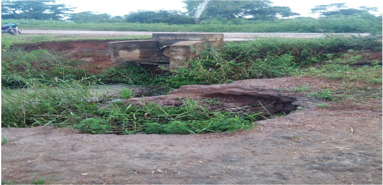
Plate 5: A typical example of gully hazard where a bridge is about to collapse at Mugau 2
